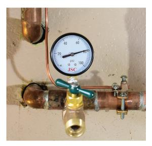
**Figure 8** - Copper wire clamped to incoming water main
