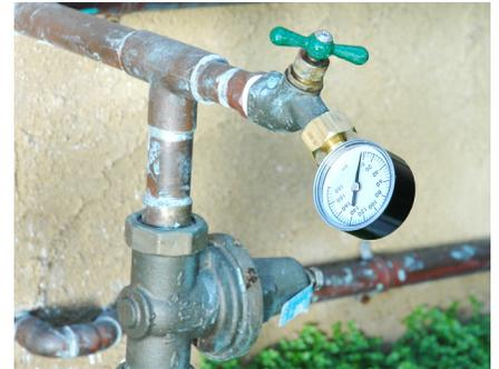
Figure 1 - Water Pressure Gauge
