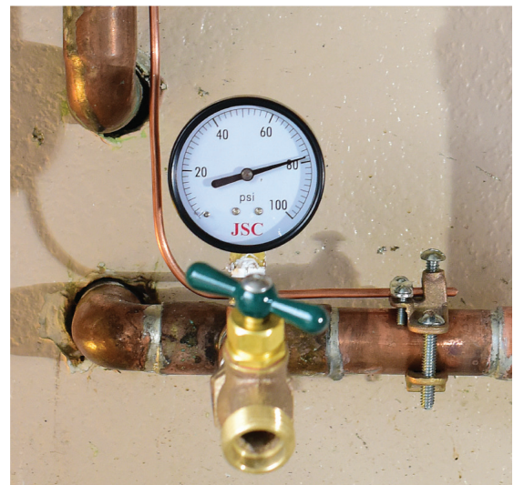
Figure 10 - Copper wire clamped to incoming water main.
