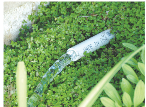
Figure 5 - System Rinse Line
