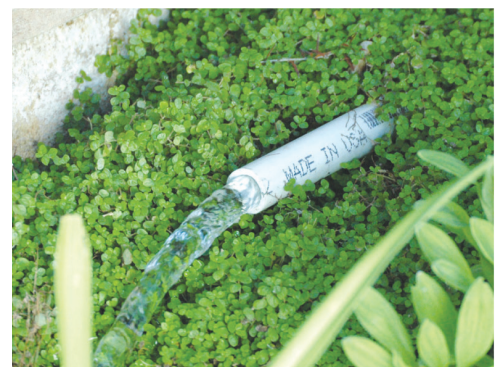
Figure 4 - System Rinse Line
