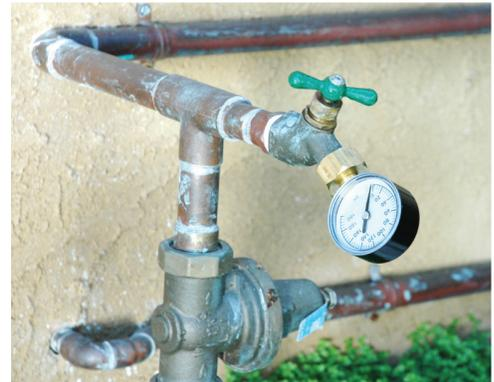
Figure 4 - Water Pressure Gauge
