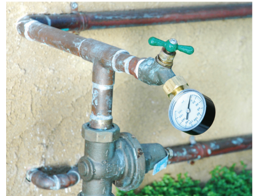
Figure 3 - Water Pressure Gauge
