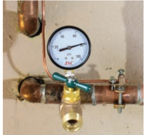
Figure 8 - Copper wire clamped to incoming water main
