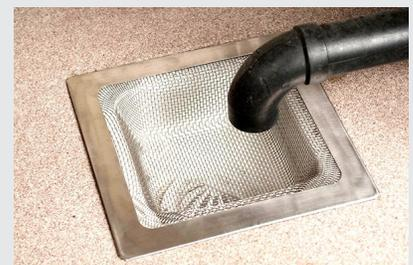
Figure 7 - Rinse line to drain.
